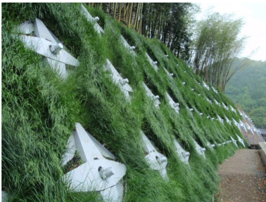
Stabilization of slopes against landslides using plant growth in Kyoto, Japan
